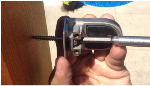
Drilling Straight-Run Connector into post
