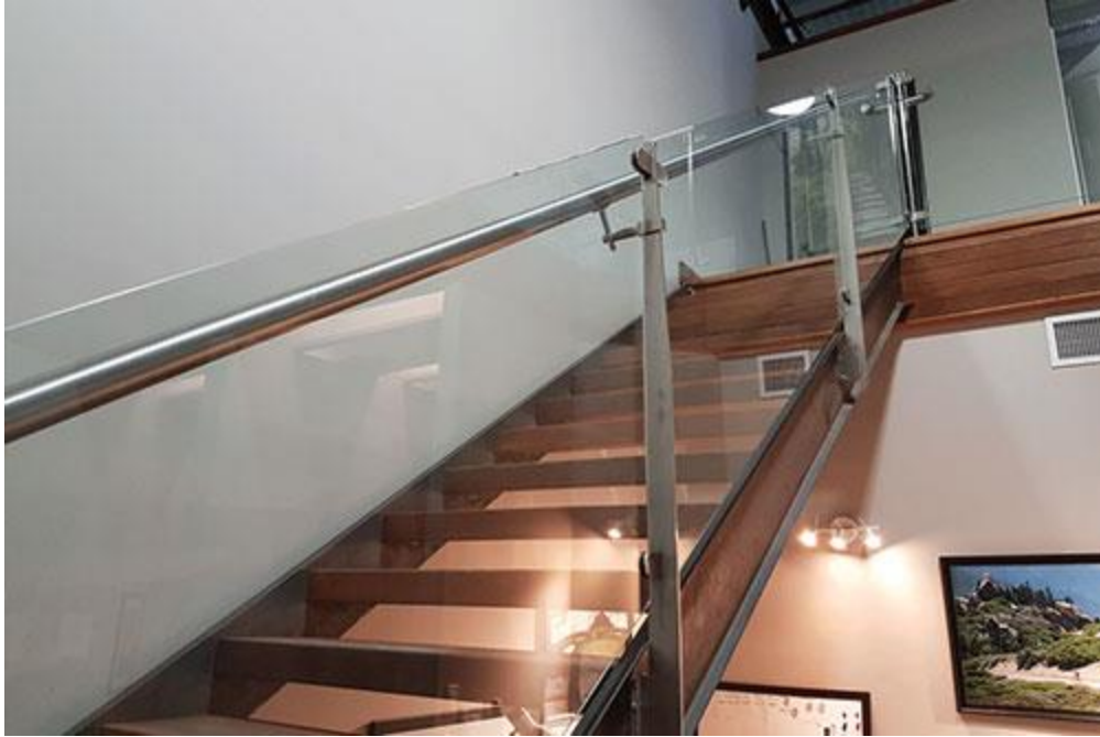
SS Invisipost mounted handrail brackets supporting SS handrail.
