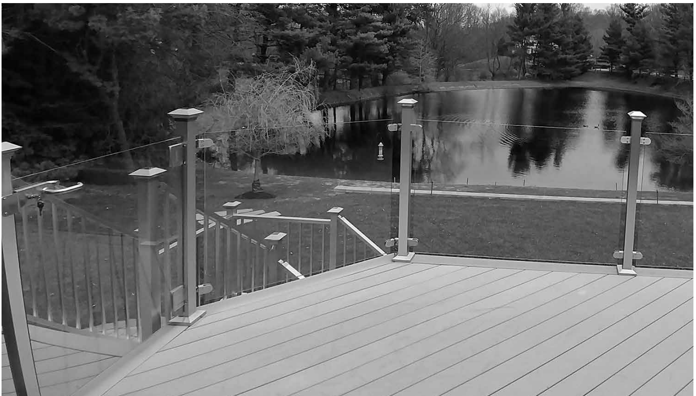
ALX post -- outside 45° w/ 45-degree bracket
